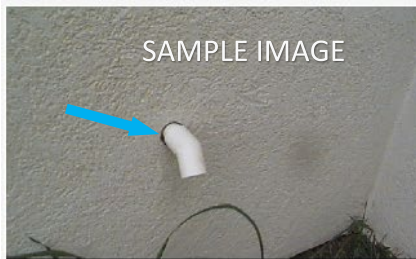
Fig. 1 Unsealed penetration
