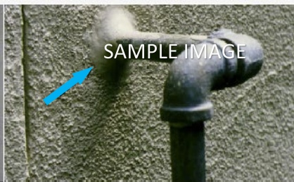
Fig. 2 Sealed pipe penetration
