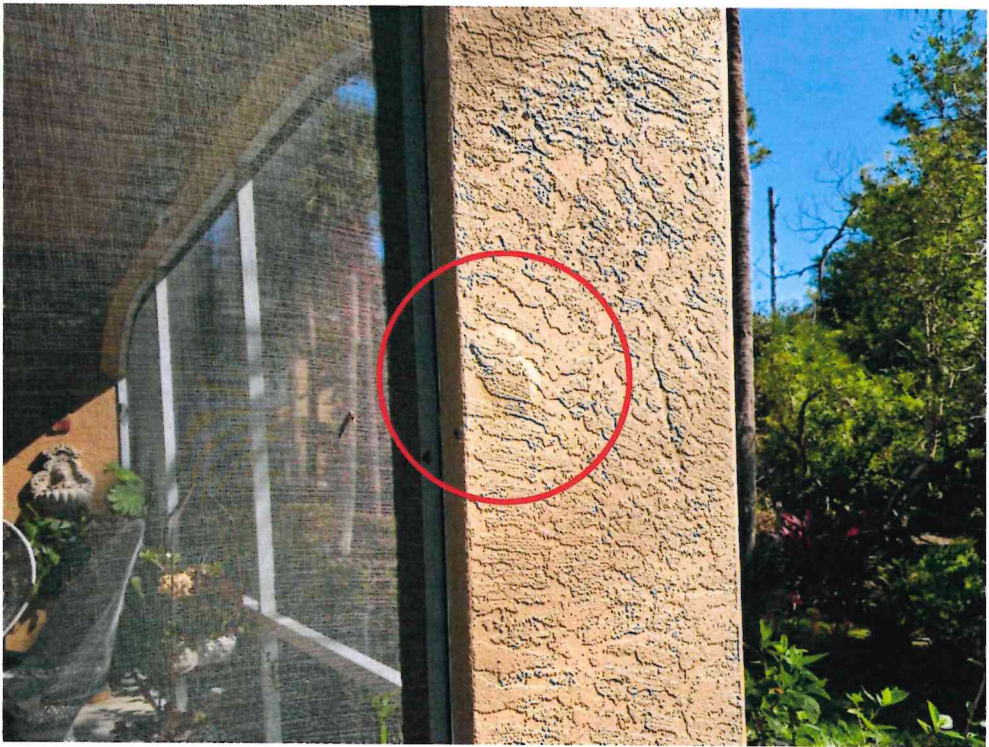
Unit 22965 – Stucco delamination on lanai column
