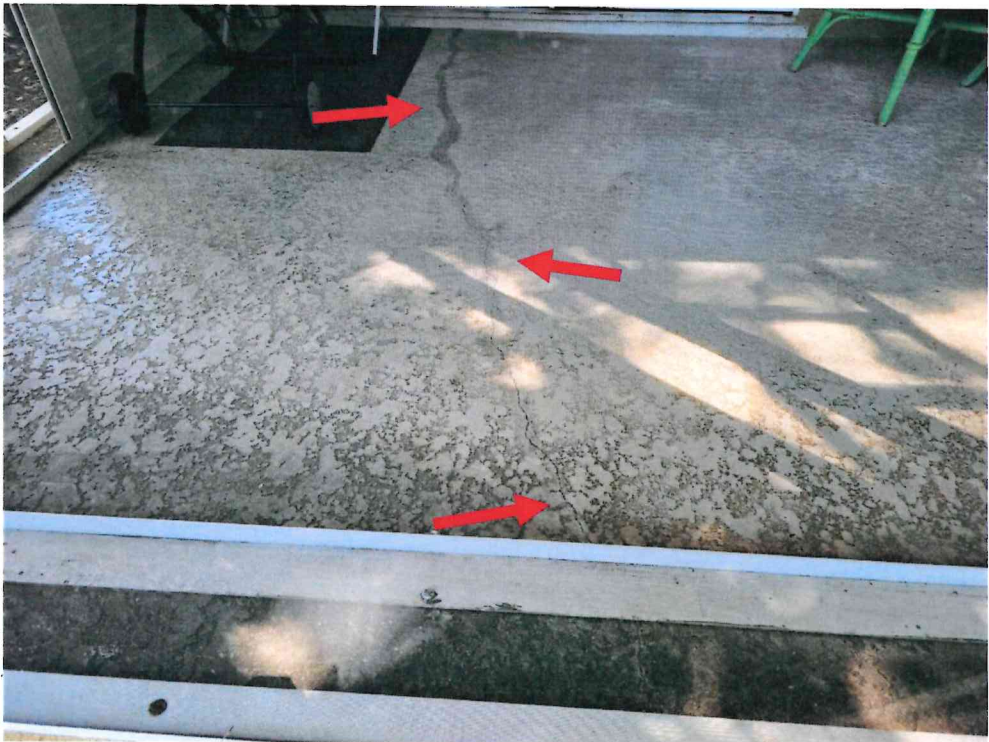
Unit 22944 – Typical crack in lanai ground floor slab
