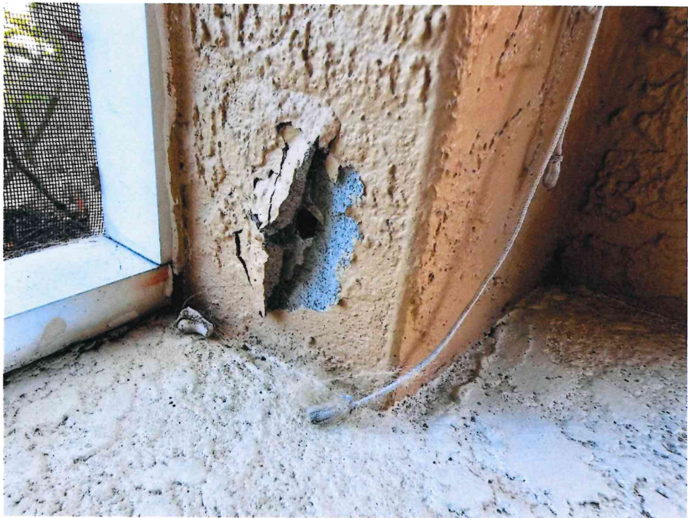
Unit 22974 – Stucco cracking and delamination on lanai column
