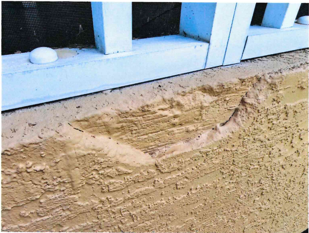
Unit 22906 – Missing and delaminated stucco on lanai slab edge
