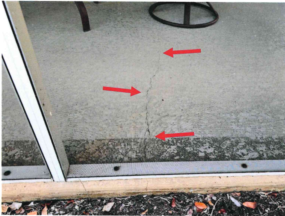
Unit 22993 – Typical crack in lanai ground floor slab
