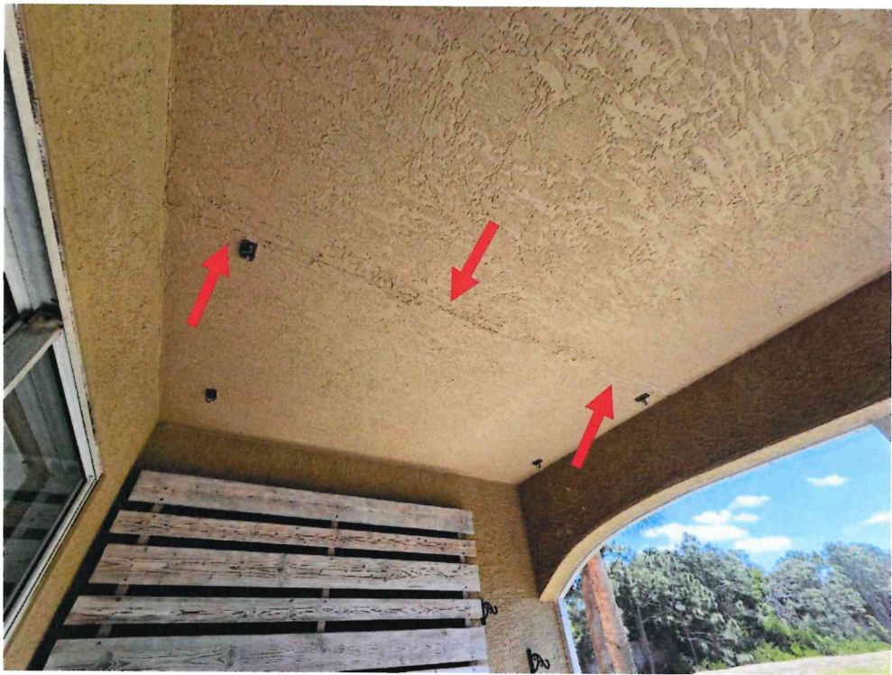
Unit 23084 – Stucco cracking on lanai ceiling along slab joint
